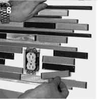
6. Once the mosaic tile installation is completed, it may be necessary to install an electrical box extender (found at your local hardware store) around electrical sockets or switches to allow the electrical plate to sit flush against the tile. **Ensure that the power supply to the outlet is turned off** when installing an electrical box extender, and follow the manufacturer's installation instructions or consult your local electrician.
